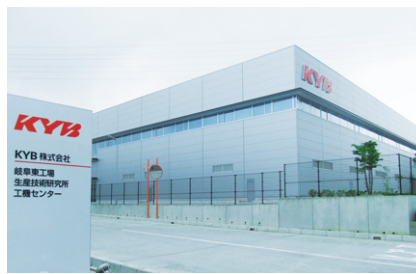
Gifu East Plant
