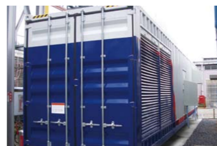
Updated cogeneration facility
