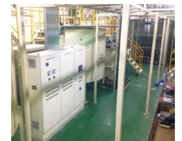
Part of the wastewater treatment installation
