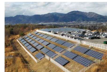
View of solar panel installation
