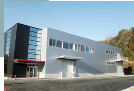
Appearance of the electronic experiment building
