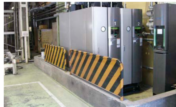
Efficient boilers for the coating system
