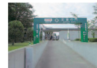
Gateway to safety erected at the Gifu North Plant
