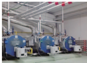
KAMS steam equipment
