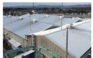
Roof after Implementation of Heat Shield Coating
