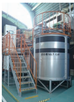
Installed Treatment Unit
