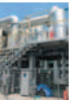
Installation of cogeneration system by ESCO operation
