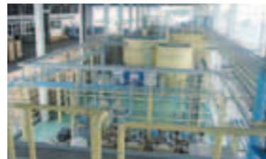
Wastewater purification process facility
