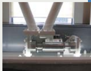
Vibration control damper
