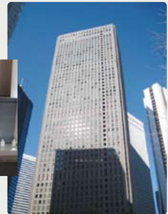
Shinjuku Center Building
