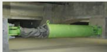
Vibration-control oil damper
