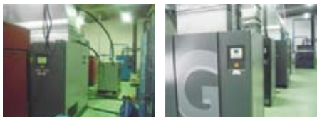
Past compressor room New compressor room
