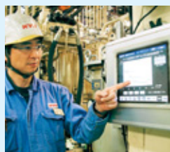
Reducing power waste by making equipment power use visible ▶
