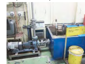
Biomass decomposition equipment
