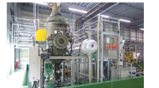
Volume reduction equipment for waste fluid in Gifu East Plant
