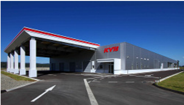
No. 2 Plant (Dedicated plant for vehicle-use ECUs)
