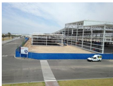
SA plant under construction (May 2015)
