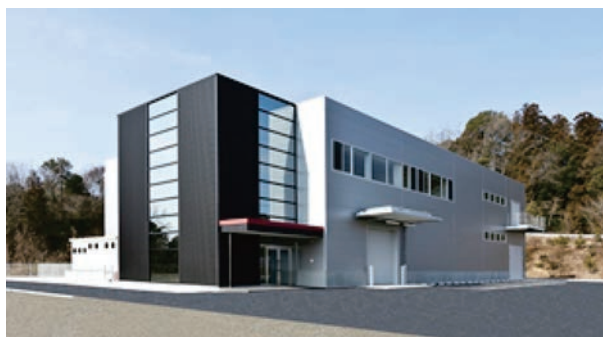
Photo 3 Appearance of Electronic Experiment Building
