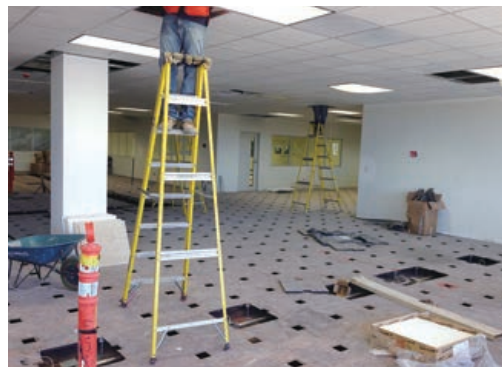
Photo 3 KMEX office under construction
