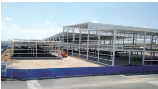
Photo 7 SA plant under construction
