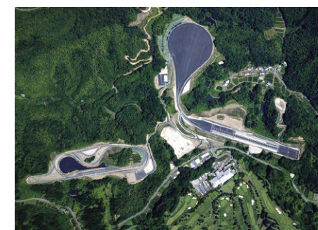
Opened the Developmental Experiment Center; began operations on the test track
