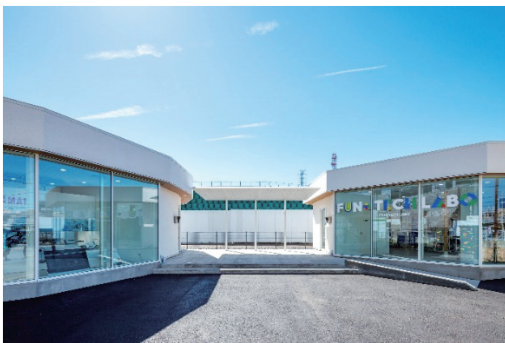
Photo 1 Exterior of FUN+TECH LABO (photo courtesy of JR Central)
