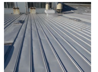
After applying heat-shield coating
