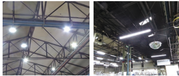
LED light devices in the high ceiling
