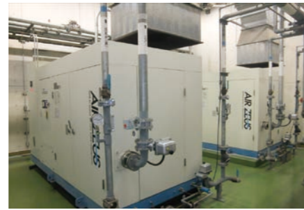
Before applying heat-shielding coating
