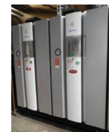
Small once-through boilers in general
