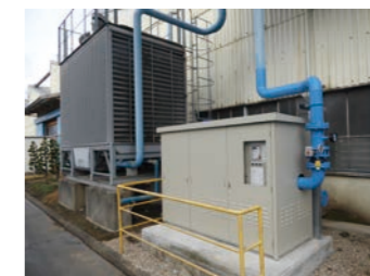
Applying inverter control for cooling towers
