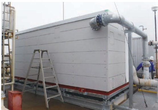
Gifu North Plant Bldg. A: Gas Burning Absorption Type Water Heater and Cooler for Air Conditioning
