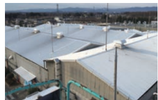
Roof after Implementation of Heat Shield Coating
