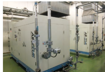
Before applying heat-shielding coating
