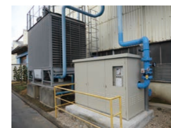
Applying inverter control for cooling towers
