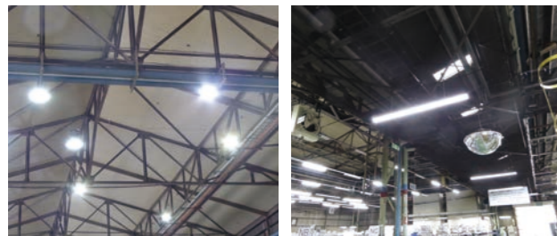
LED light devices in the high ceiling
