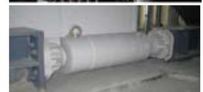
Tokyo Mode Gakuen and 110 units of 2000kN vibration control oil dampers
