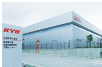
Gifu East Plant
