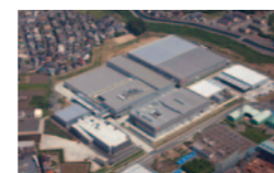
Gifu East Plant
