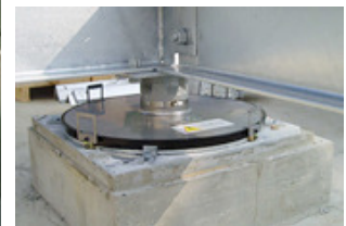
Ball isolator for home base isolation
