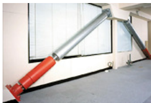
Building vibration control
