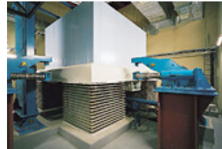
AMD building vibration control device
