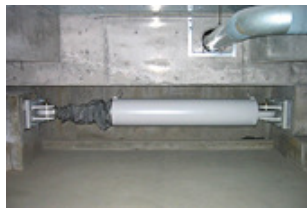
Building base isolation
