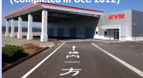
KYB Trondule No. 2 Plant at Niigata pref. (Completed in Oct. 2012)
