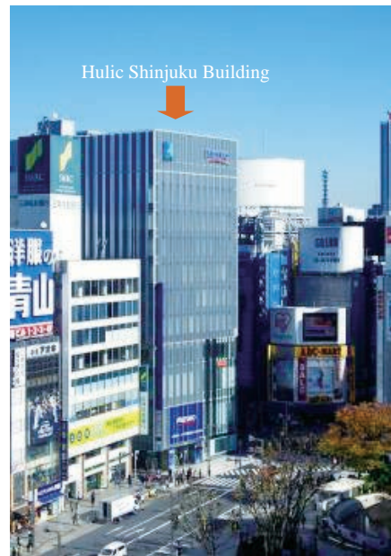
Photo 4 Hulic Shinjuku Building appearance
