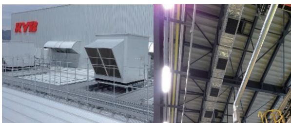
Photo 7 Air supply system outside and inside the plant
