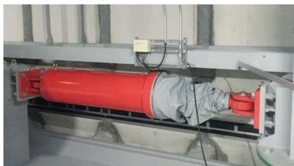
Photo 2 Installation example of the oil damper with a lock mechanism
