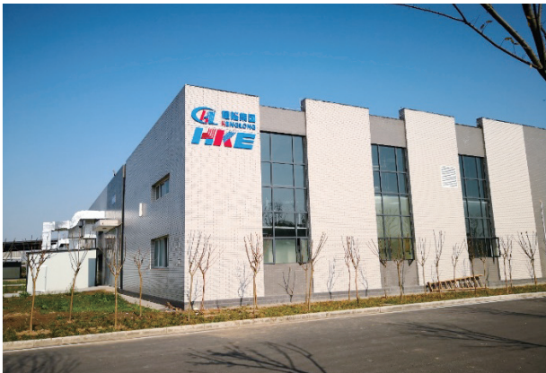
Photo 1 Appearance of HKE building
