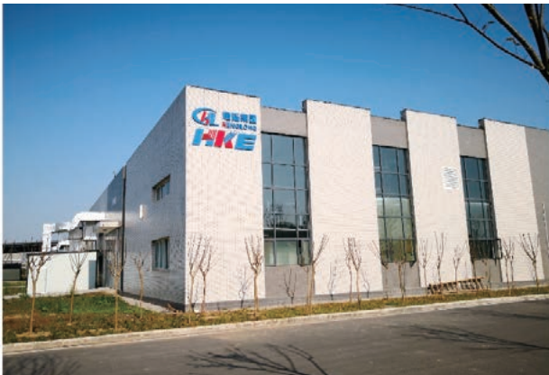
Photo 1 Appearance of HKE building
