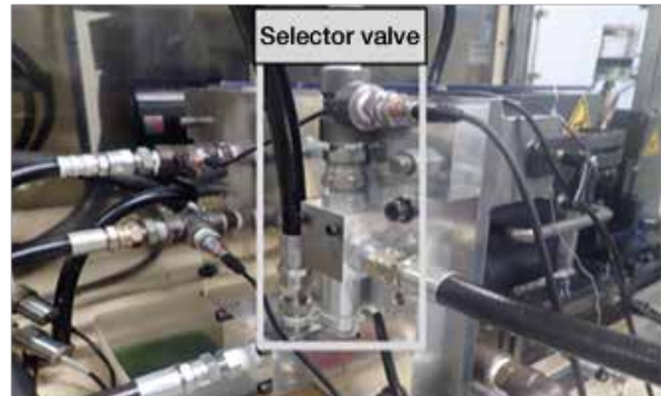
Photo 1 Valve change-over test machine
