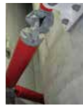
High-speed Oil Dampers 高速油缓冲器 They have been installed in the TOKYO SKYTREE® as vibration control devices. 用于东京晴空塔的抗震装置。
