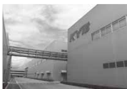
Gifu East Plant
