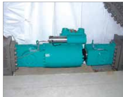
制振ダンパ Building Vibration Oil Damper
