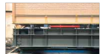
戸建住宅免震装置 Earthquake Isolation Device for Detached House
