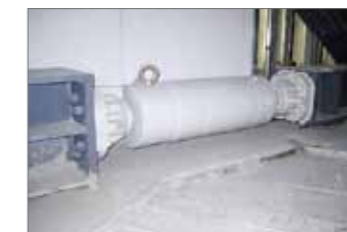
200t制震ダンパ 200t Type Oil Dampers for Vibration Control Devices
