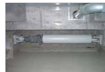
ビル免震用オイルダンパ Oil Dampers for Basic Isolation of Buildings
